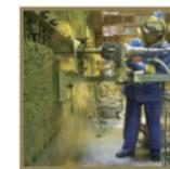
Installation method of large scale reinforcing anchor bars by water jet drilling
